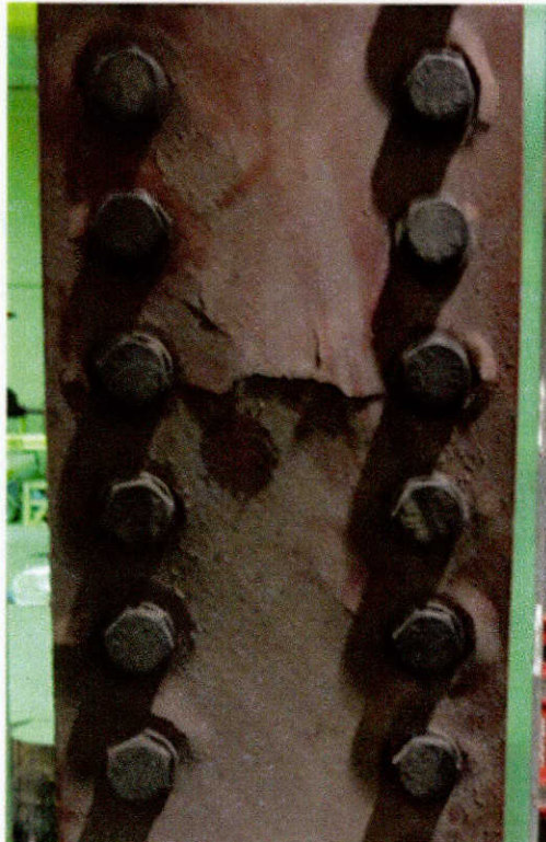
Figure 10.34: Global buckling of the piles repaired with Repair System 3
