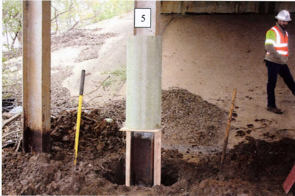
(a) Positioning of GFRP jacket on pile 5
