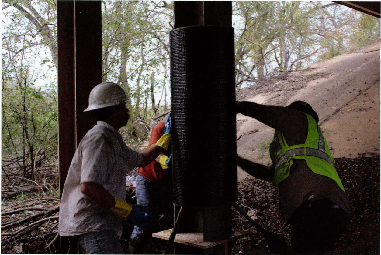
Figure 12.7: Installation of the CFRP overwrap
