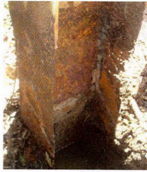
(a) Reduction of Flange Width
