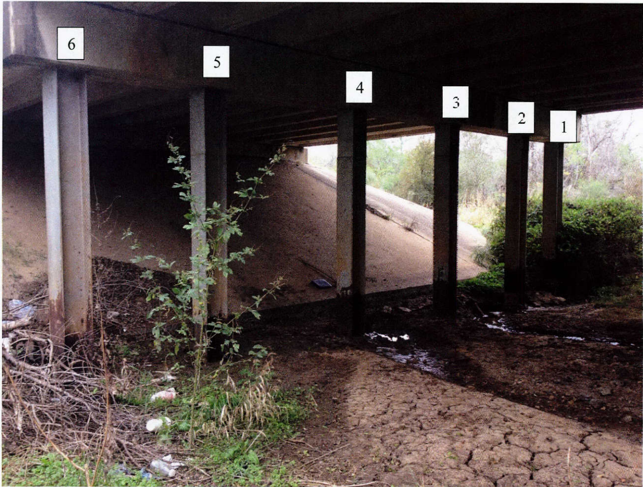
Figure 12.3: Site conditions on November 30, 2015
