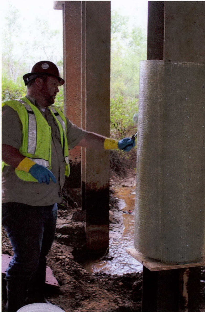
Figure 12.6: Coating the GFRP jacket with epoxy
