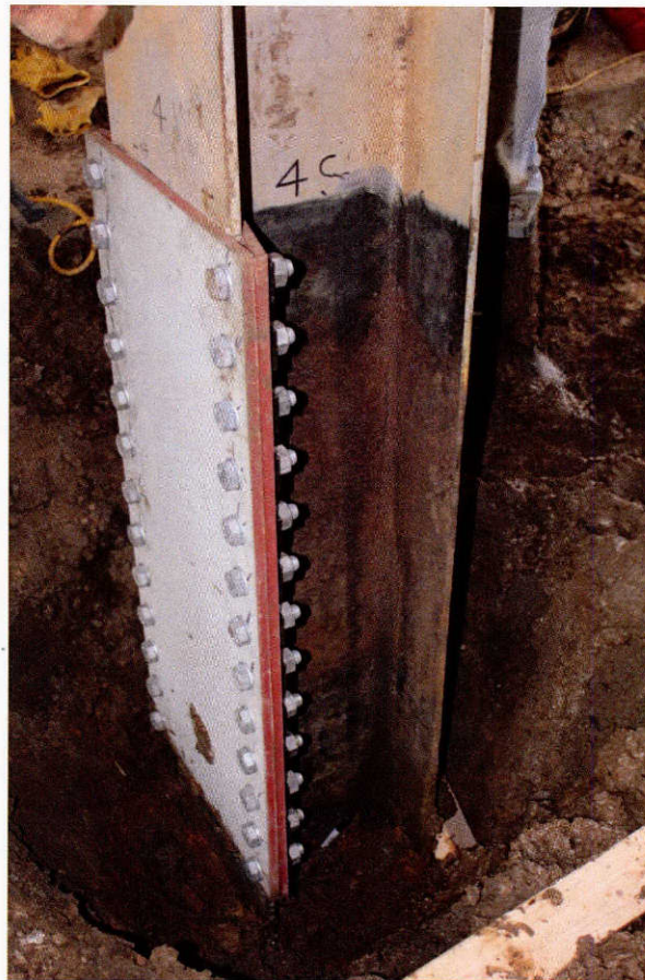
Figure 12.12: Steel based repair system
