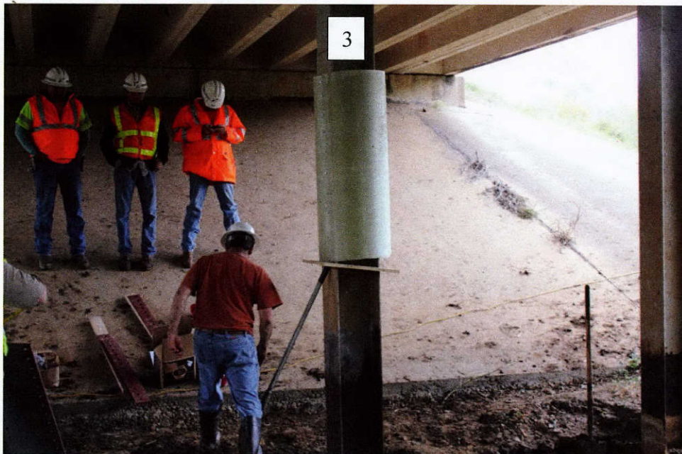
(b) Positioning of GFRP jacket on pile 3
