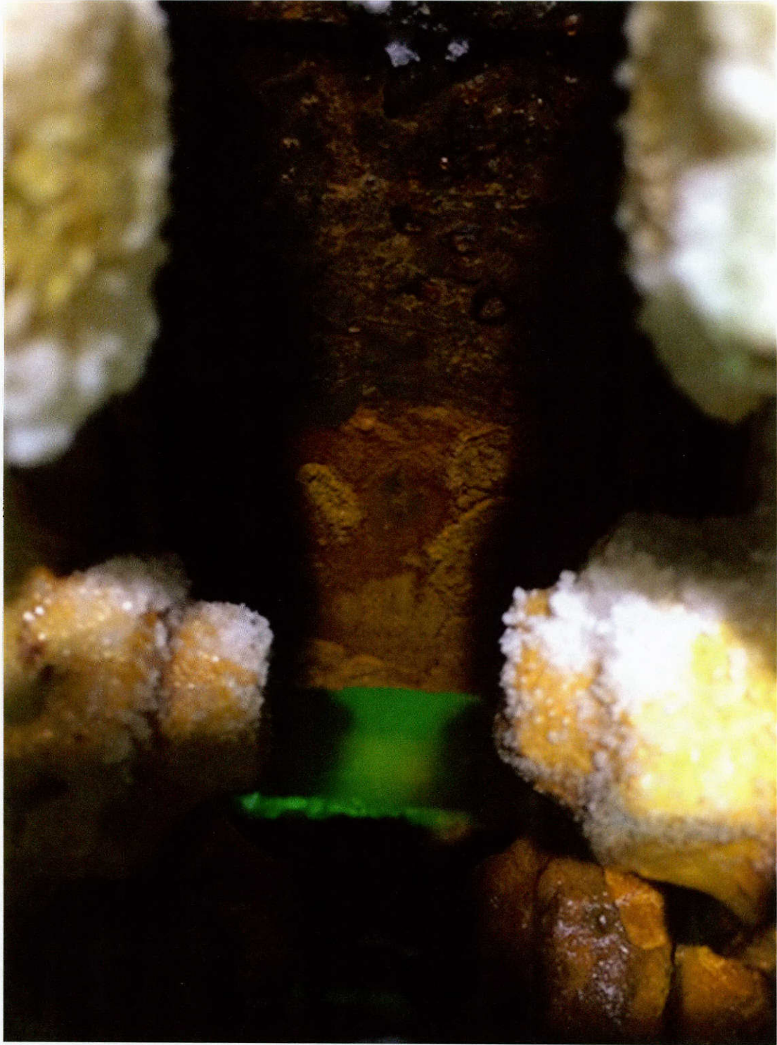
Figure 10.48: Web and bolt corrosion for Repair System 3 (S3-12-Cor)
