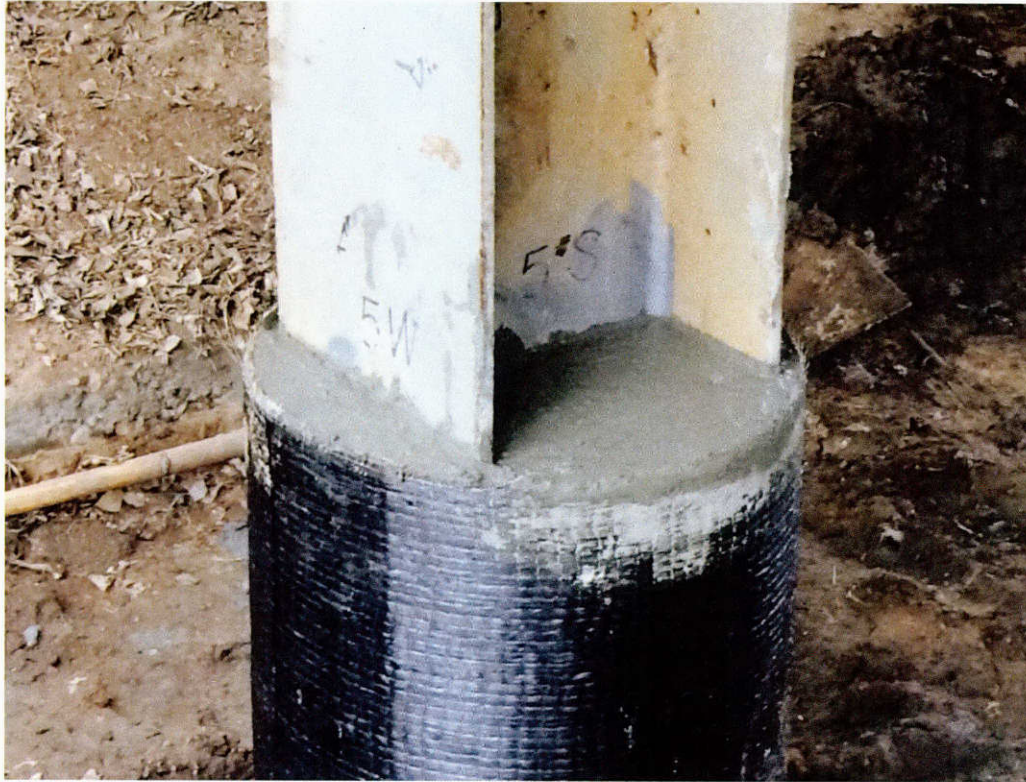
Figure 12.8: Completed installation of grouted FRP-jacket
