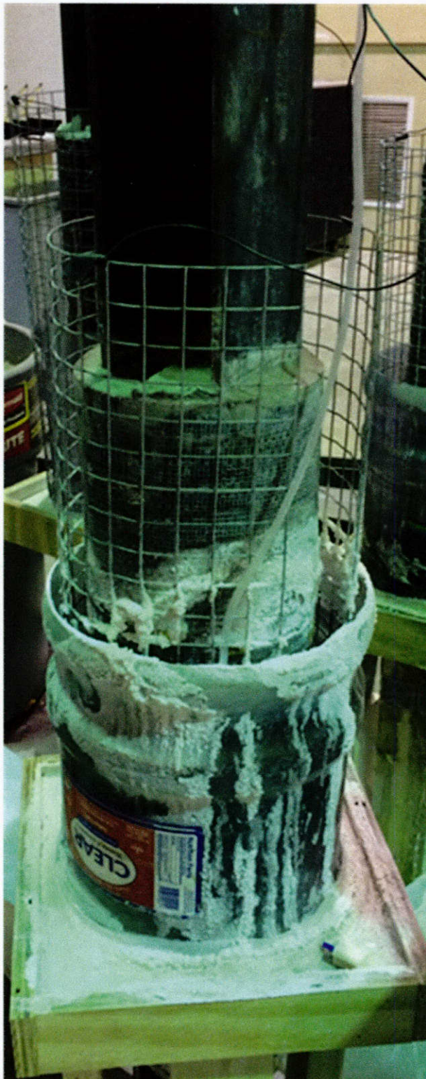
Figure 10.42: A damaged pile repaired with Repair System 1 (S1-4-Cor) showing no evidence of corrosion
