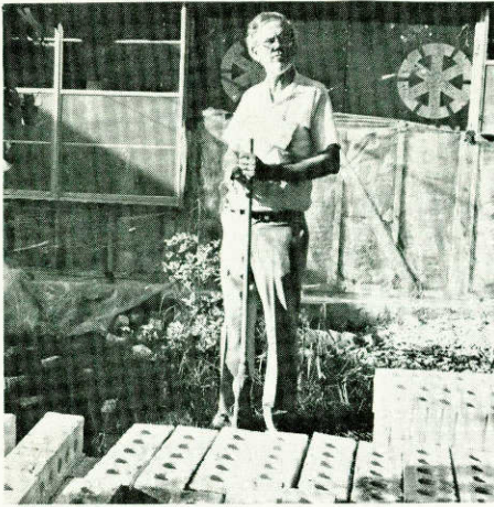
The brick on the back of Program Specialist Don May's home was knocked off by a car that was slammed into the wall by swirling flood waters. The May family received part of the Austin TRC Flood Victim Fund.
