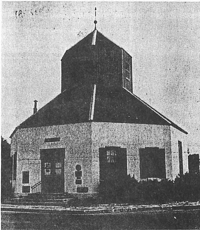
ONE OF THE CITY'S most uniquely-shaped structures is the Vereins Kirche, located in the heart of the city on Market Square. Completed in 1935, the replica of the original Vereins Kirche houses the Gillespie County Historical Society's "Archives Collection". —Standard-Radio Post Photo
