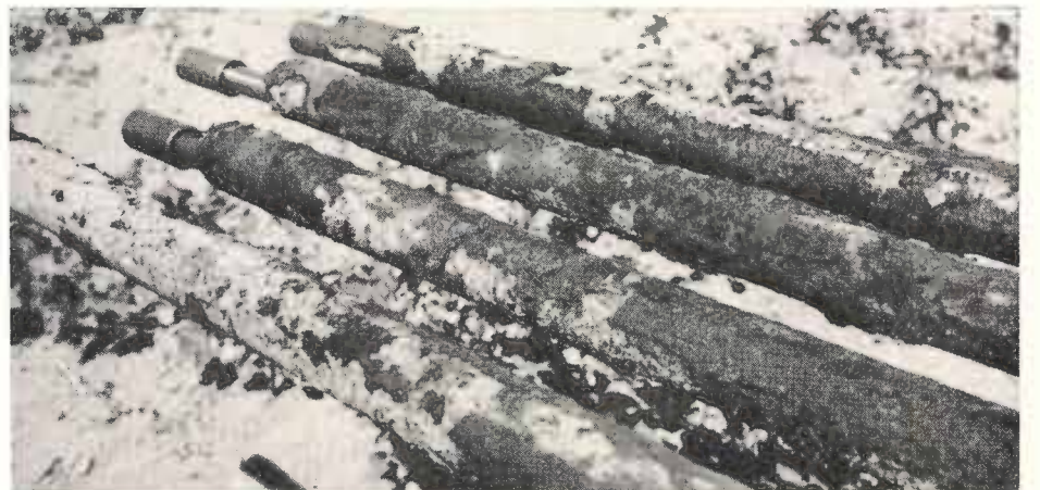
Pictured above are irrigation well oil tubes covered with an algae or bacteria growth. The growth has been found in several wells and represents a potential threat to continued normal pump operation.
