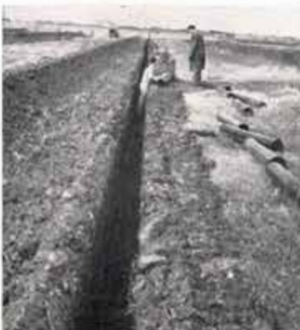
Picture shows ditches that were cut across the bottom of the lake. Various backfill materials were used to cover the lateral lines. Rainfall that collects in the lake will filter through the backfill material and enter the lateral system through openings in the wall of the pipes. Tech Photo.
