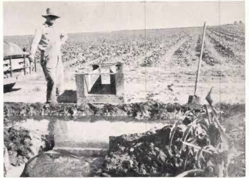
Rectangular Weir and Parshall flume used to measure discharge from the irrigation ditch to the field.
