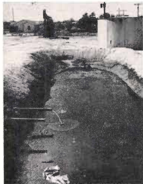
Salt water that is pumped with oil from far beneath the earth's surface, has in the past been disposed of in earthen pits. The Water District passed rules forbidding this type of disposal when it was discovered that the salt water was percolating from the pits to the fresh underground water.
