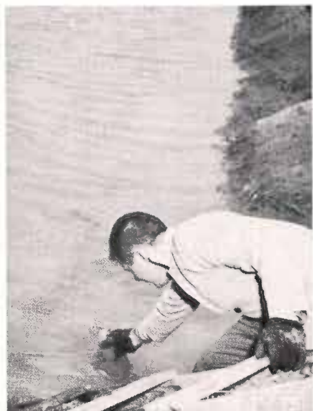
Periodic samples are gathered from the pit to determine the effectiveness of chemical reaction on the particles of silt and clay suspended in the lake water.
