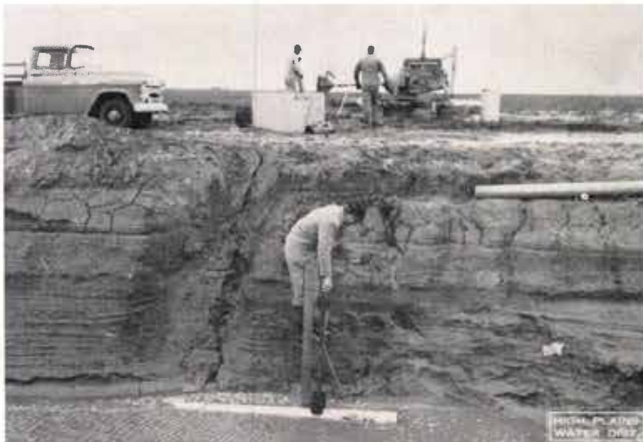
An adjustable pipe serves as an intake to the recharge well from the pit. Water is taken from the pit near the surface in an effort to draw into the well a minimum number of flocculating particles, which might remain in suspension.
