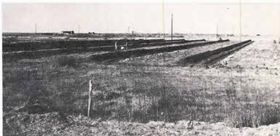
Picture shows ditches that were cut across the bottom of the lake. Various backfill materials were used to cover the lateral lines. Rainfall that collects in the lake will filter through the backfill material and enter the lateral system through openings in the wall of the pipes. Tech Photo.
