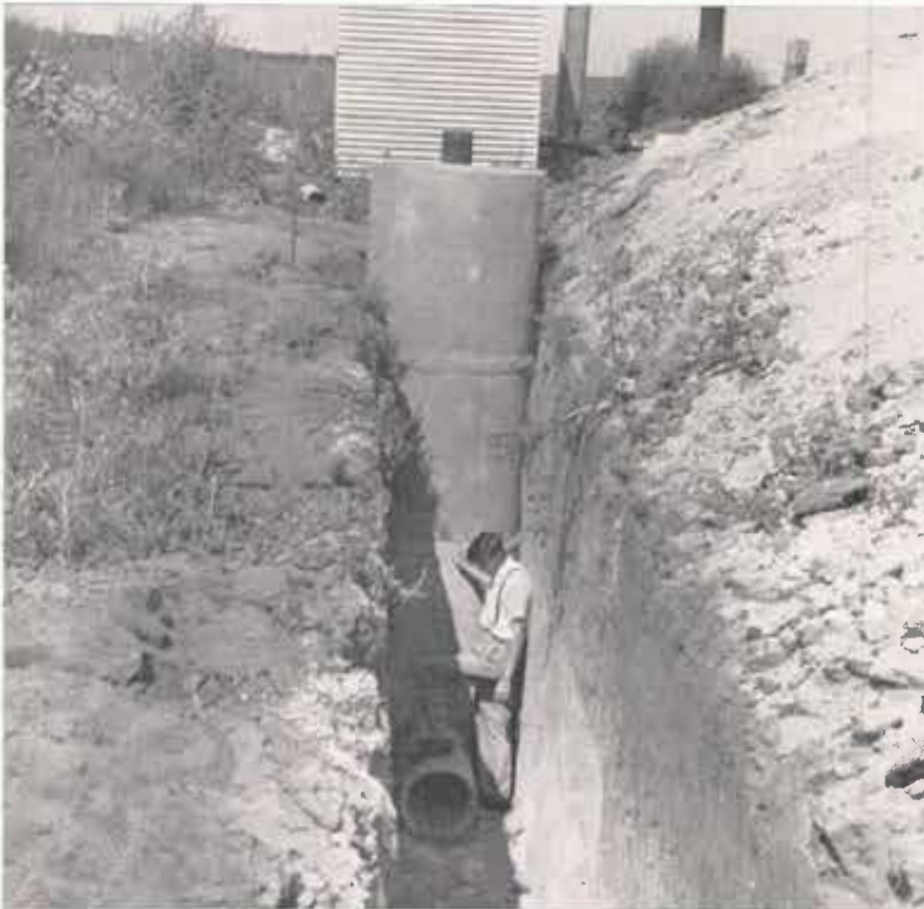
The 36-inch concrete main-line metering station is shown above. Note that the main line, which transports water gathered from the lateral lines to the meter station, had not been connected at the time the picture was made. A flow-meter built into the meter station records the quantity of water entering the recharge well from the system. Tech Photo.
