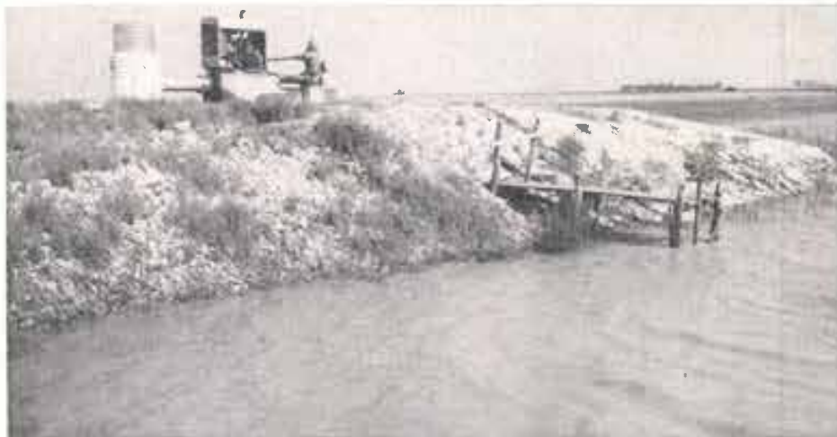
Surface water that collects in the many wet-weather lakes, under normal conditions, is mostly lost into the atmosphere by evaporation. Many multi-purpose wells (production and recharge) have been drilled near lakes in order to drain the lake water into the underground reservoir through the well.
