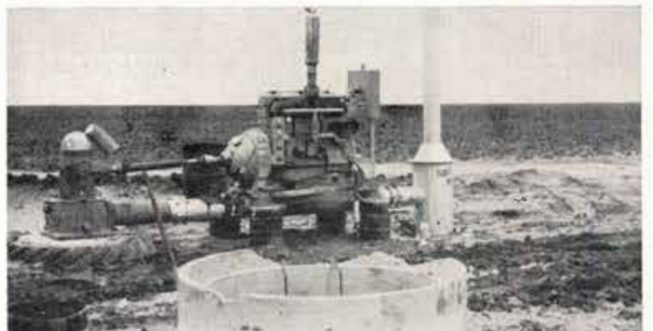
FIGURE 5—Sutton recharge well is also used as normal irrigation well.
