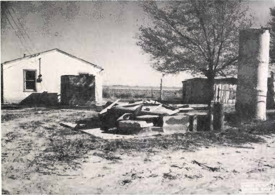
Pictured above is an abandoned well in the yard of a southern High Plains' house. It has not been properly closed—only a thin slab of concrete covers the open well shaft. Enterprising youngsters at play could remove the slab.
