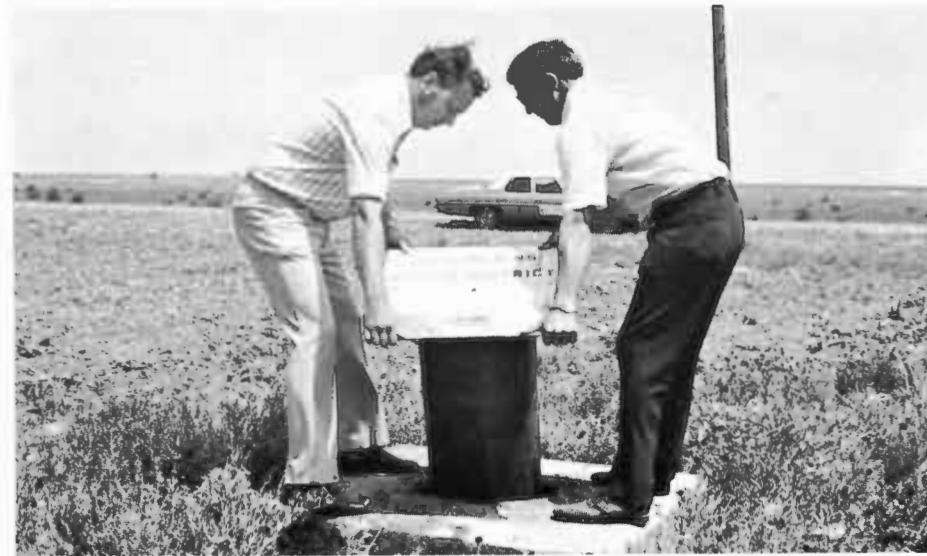
Tony Schertz and George Tull, Draftsman and Field Representative for the District, balance a steel plate welded to a piece of casing. This is a sample of an approved method of capping a well.
