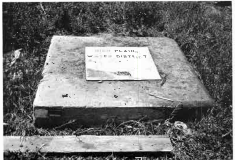
Pictured above is a view of the plug shown in the picture at left after it has been inserted into the well. The District recommends a plug of this type. (Note tire tracks of farm vehicles that have been driven over the well cover.)
