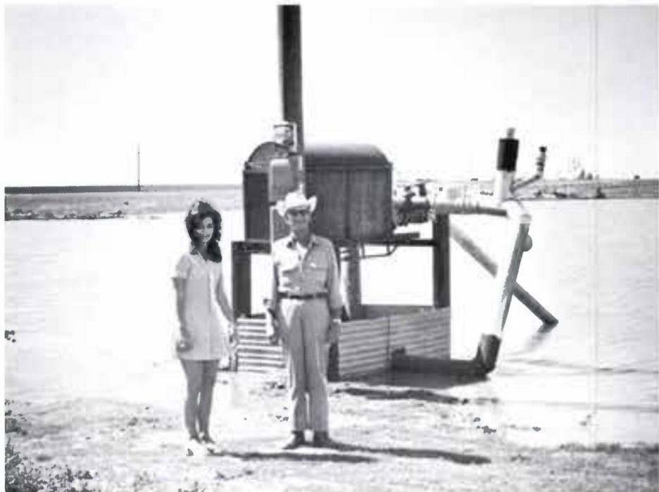
Rebecca Clinton and Tommy McKinnon stand in front of the centrifugal pump located on his playa lake he recently purchased for the purpose of irrigating his land with surface water.
