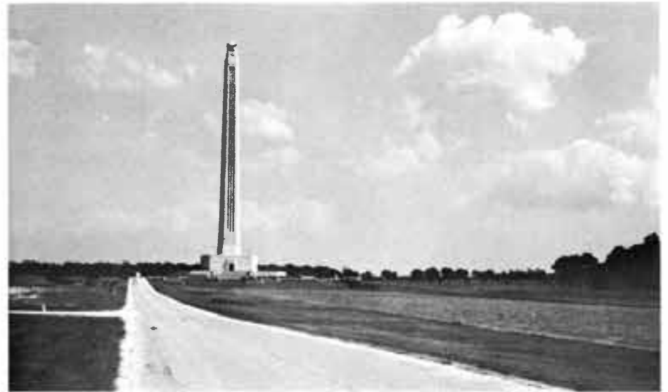
The San Jacinto monument, east of downtown Houston, is located near the area experiencing the greatest land subsidence—nearly seven feet. Land subsidence is taking place over a wide area and is sinking at a relatively even rate; therefore, the monument is not endangered, although water from Galveston Bay is encroaching upon some of the San Jacinto Park land.
