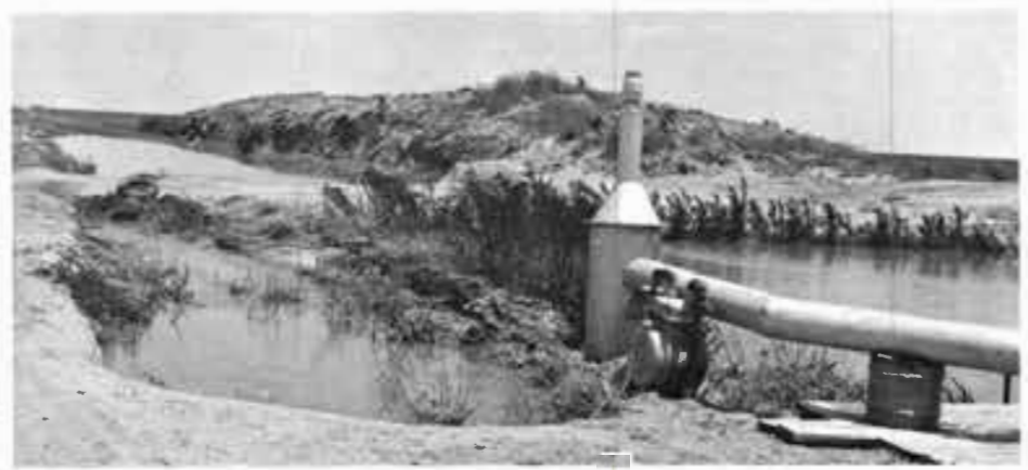
The bottom left corner of the above picture shows the ditch which carries tailwater into a silt pit (shown in the top left corner). Here the silt settles before the water flows into the tailwater pit (right portion of the picture) for redistribution.
