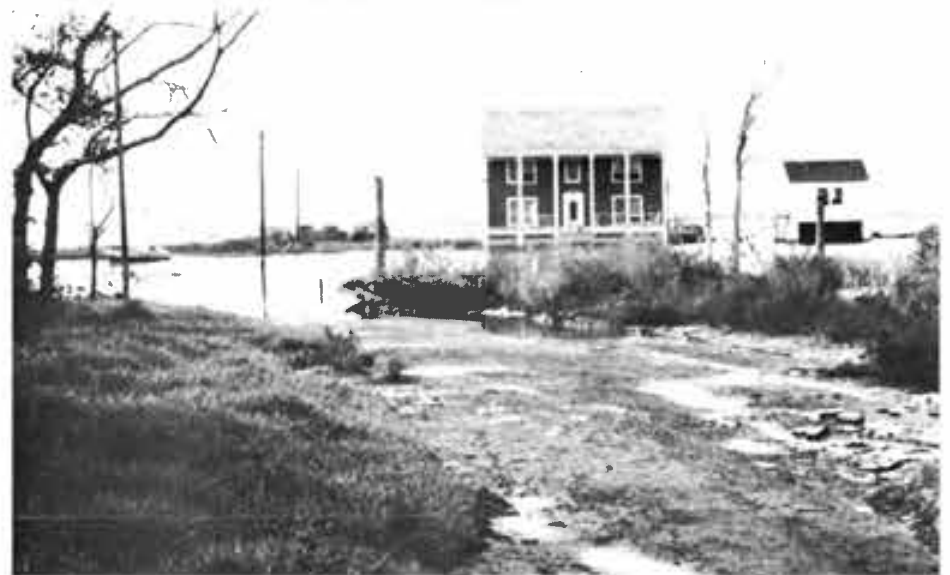
Effects of land-surface subsidence in the Houston area are indicated by the two-story home and detached garage which have been abandoned. The land surface, where the house now stands, formerly stood several feet above the water level of Galveston Bay, which now surrounds the house.
