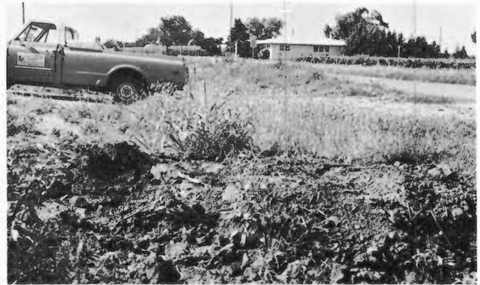
Within a week the Highway Department filled the hole with ten yards of dirt and grass. J. B. Sparks, Area Foreman for the Department, said his crew will frequently check the abandoned well for possible cave-ins, and may later plug it with a concrete slab.
