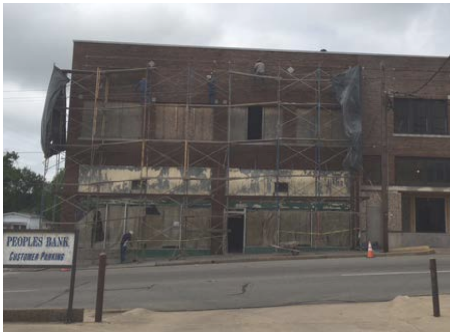
Paint removal in process at 134 1st St. SW in Paris.
