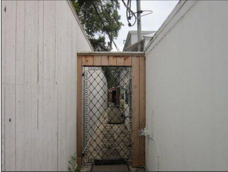
6 - Back of house (east side, looking south)
