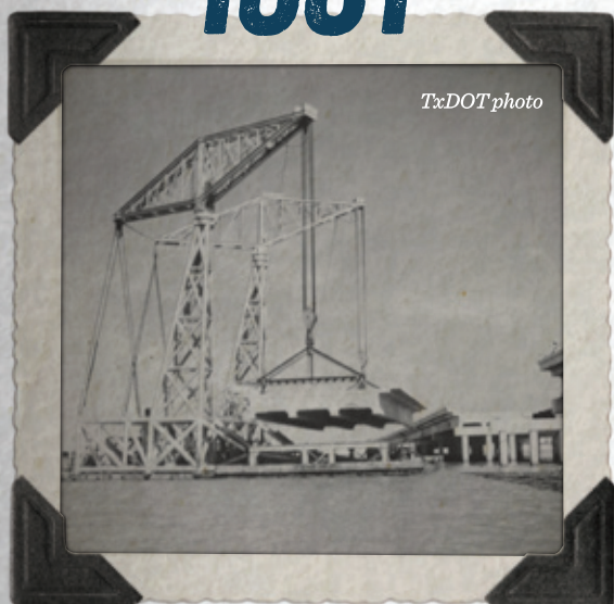
Construction in 1961 of the new Lavaca Bay Causeway in the Yoakum District.
